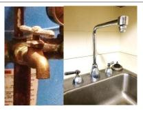
(Step 1) Find a sampling tap to draw water sample from. The pressure tank sampling tap is a good location. A kitchen tap may also be used, Do NOT use an outside tap.
